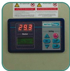
Microprocessor Control Panel
